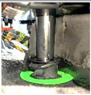
3. Here the drain hose is incorrectly installed and will require replacement to seal properly.
